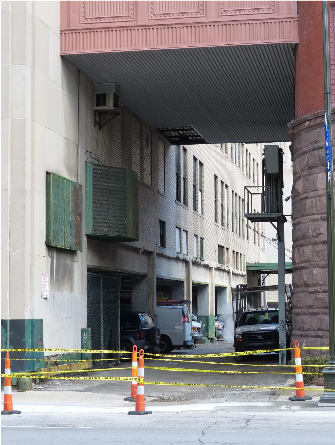
Figure #10: Exterior, Looking Northeast. 12/9/2016
