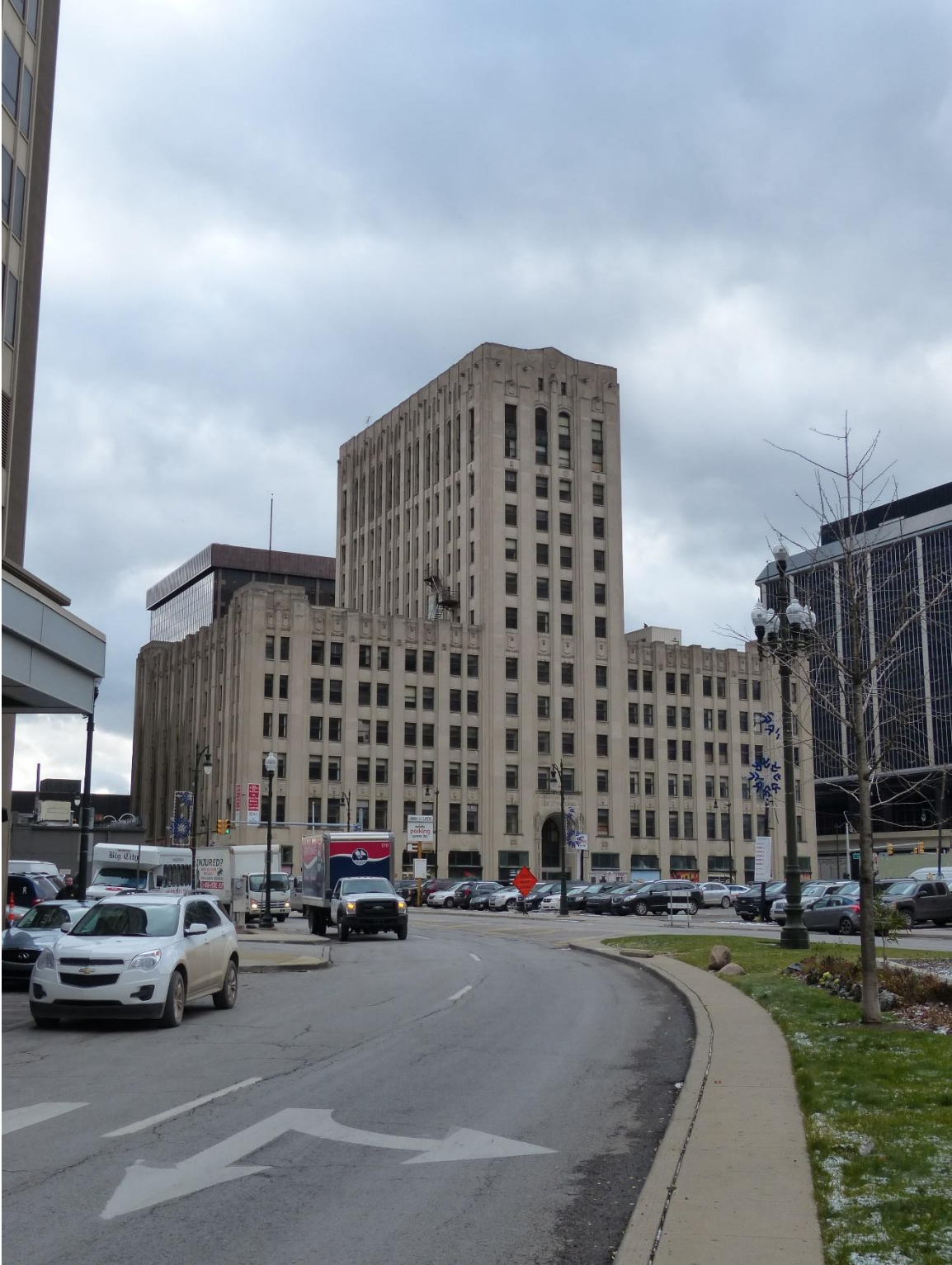
Figure #3: Exterior, Looking Southwest. 12/9/2016
