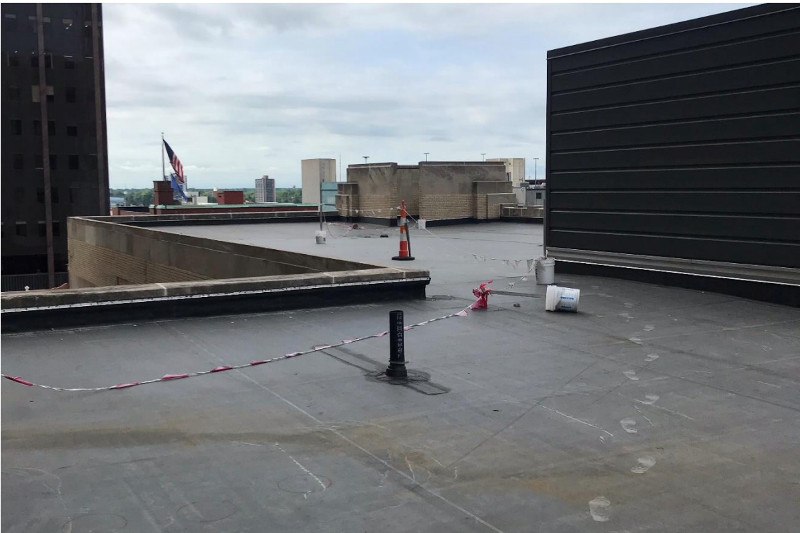
Figure #4: Exterior, West Roof, Looking Northeast. 7/31/19
