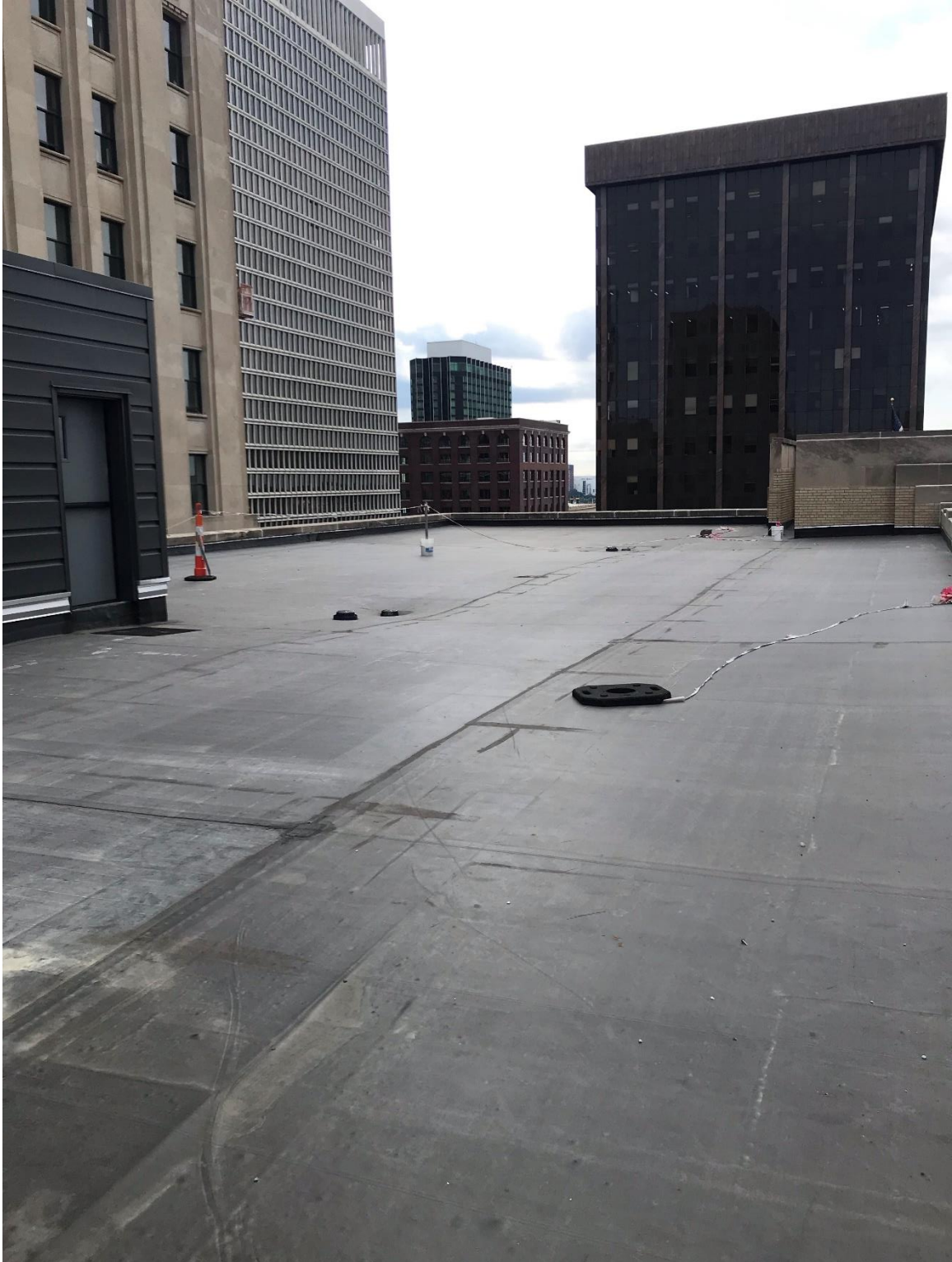
Figure #5: Exterior, West Roof, Looking South. 7/31/19
