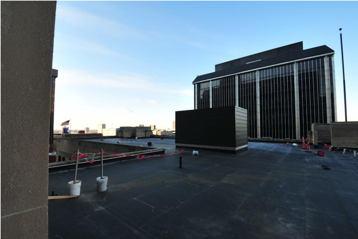
Figure #1: Exterior, West Roof, Looking Southwest. 3/11/19
