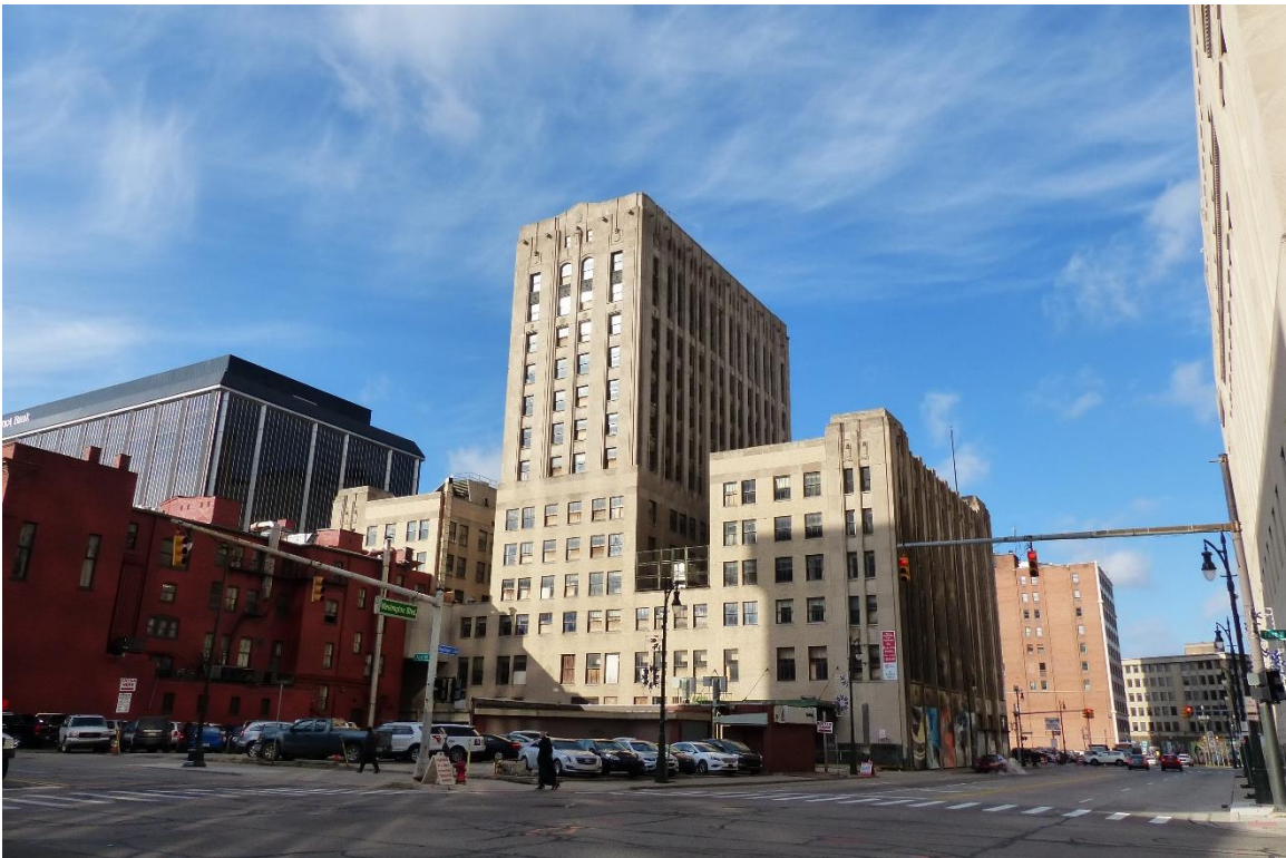
Figure #6: Exterior, Looking Northwest. 12/7/2016
