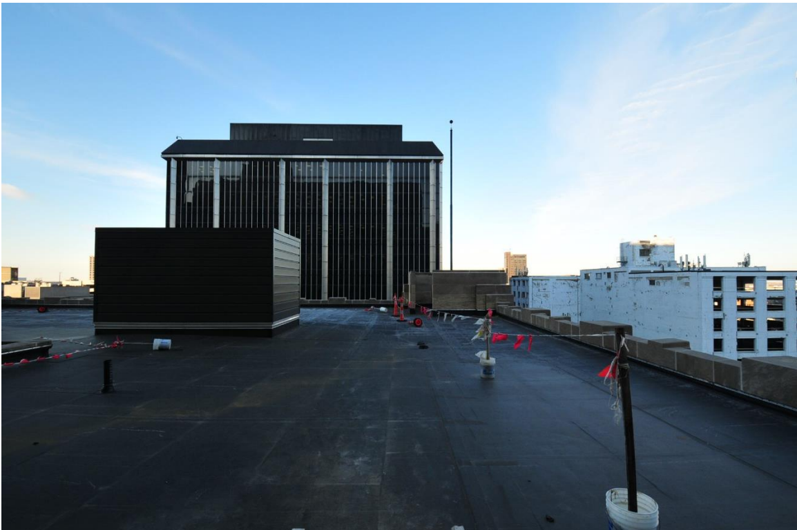
Figure #2: Exterior, West Roof, Looking West. 3/11/19
