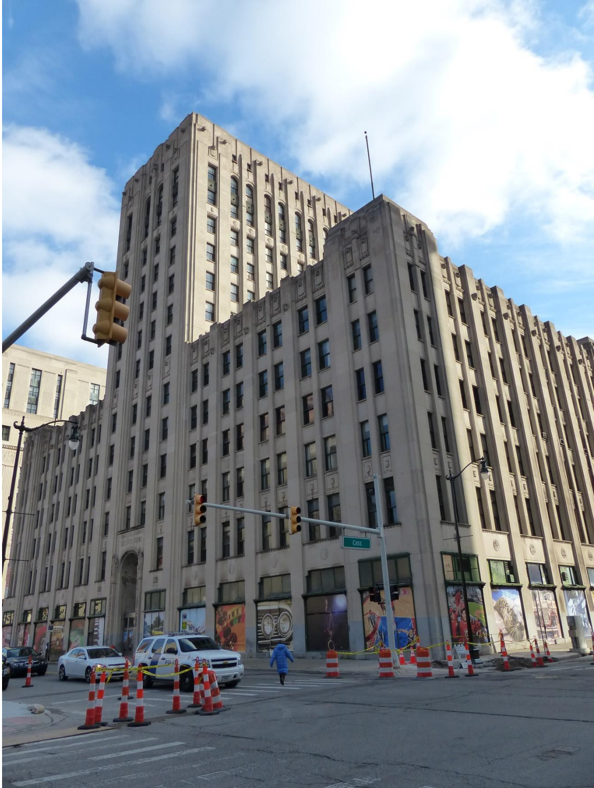
Figure #1: Exterior, Looking Southeast. 12/7/2016
