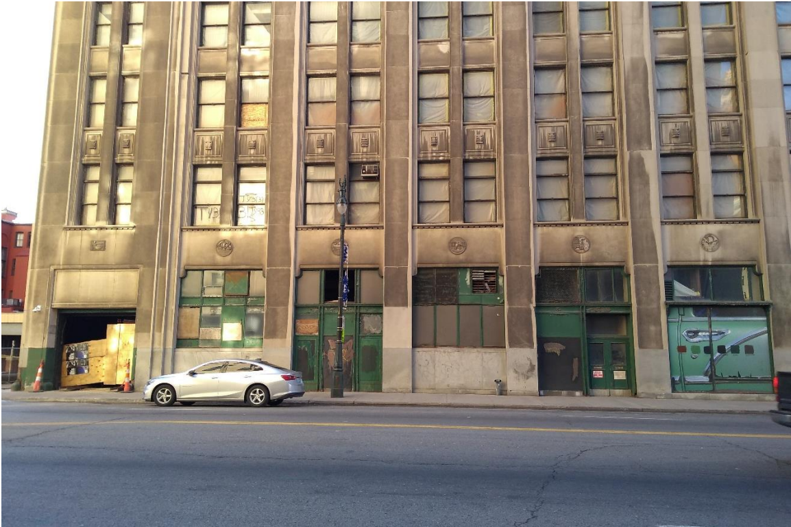
Figure #5: Exterior, Looking West. 1/30/2017
