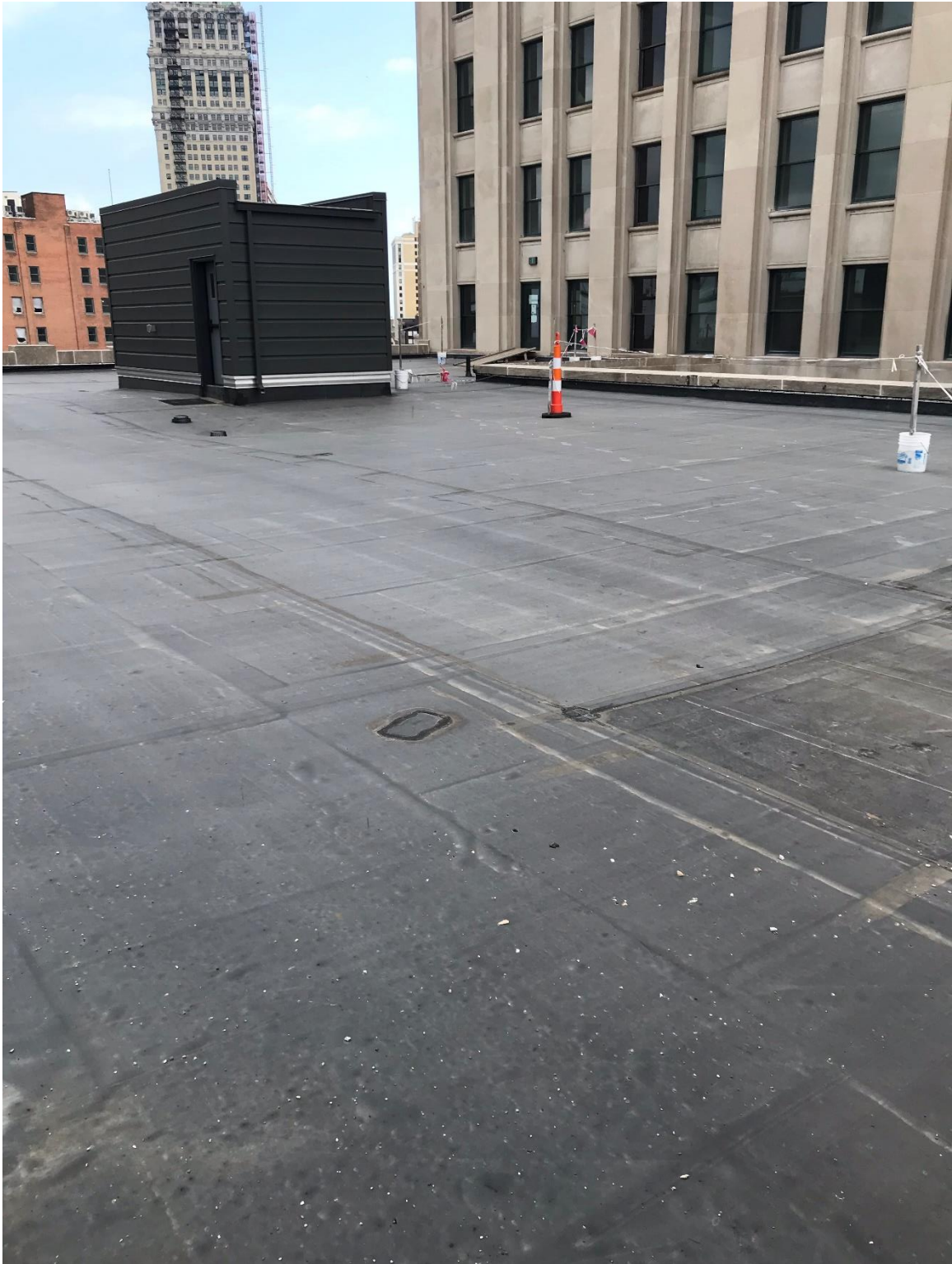
Figure #6: Exterior, West Roof, Looking Northeast. 7/31/19
