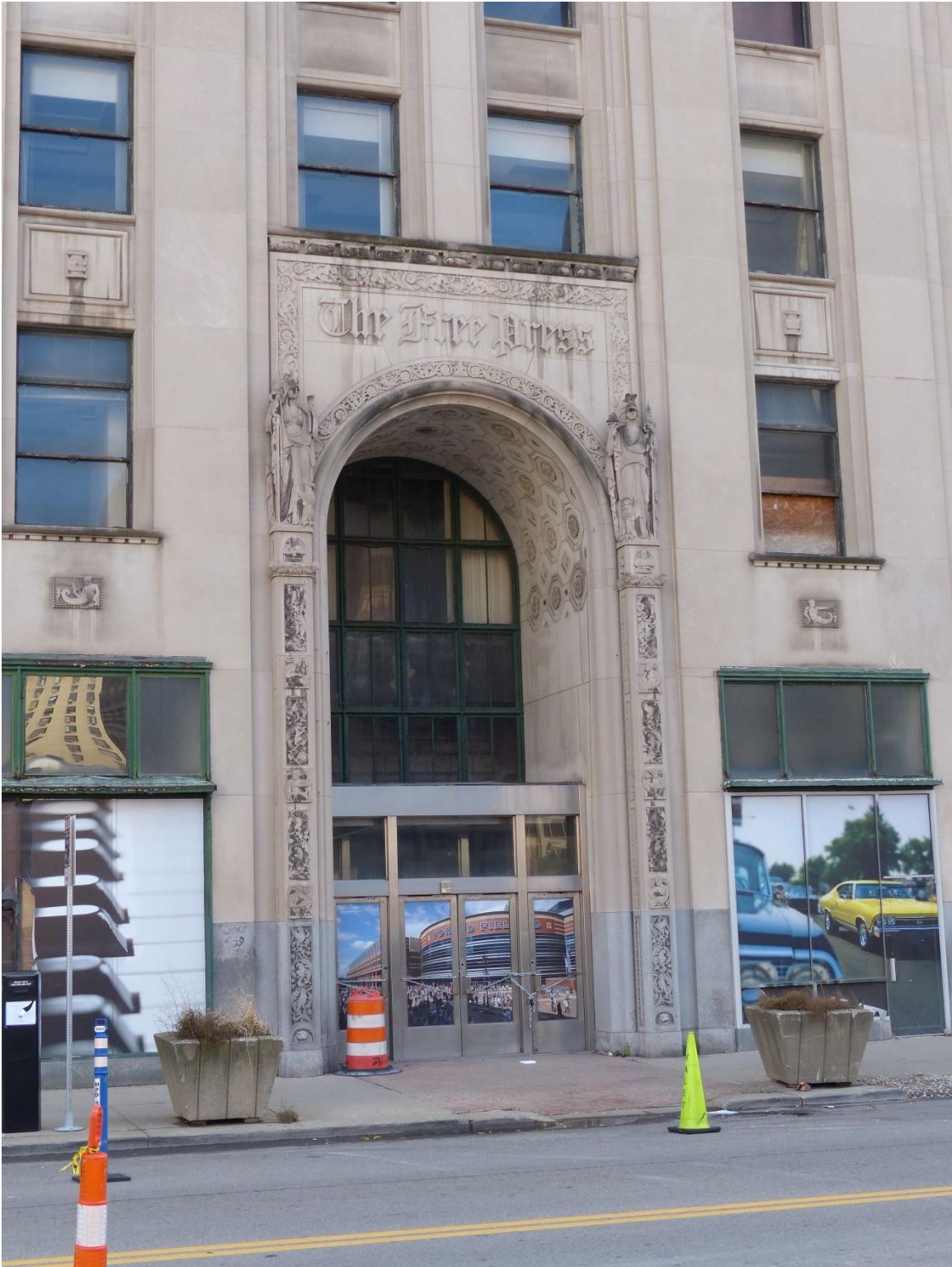
Figure #4: Exterior, Looking Southwest. 12/7/2016
