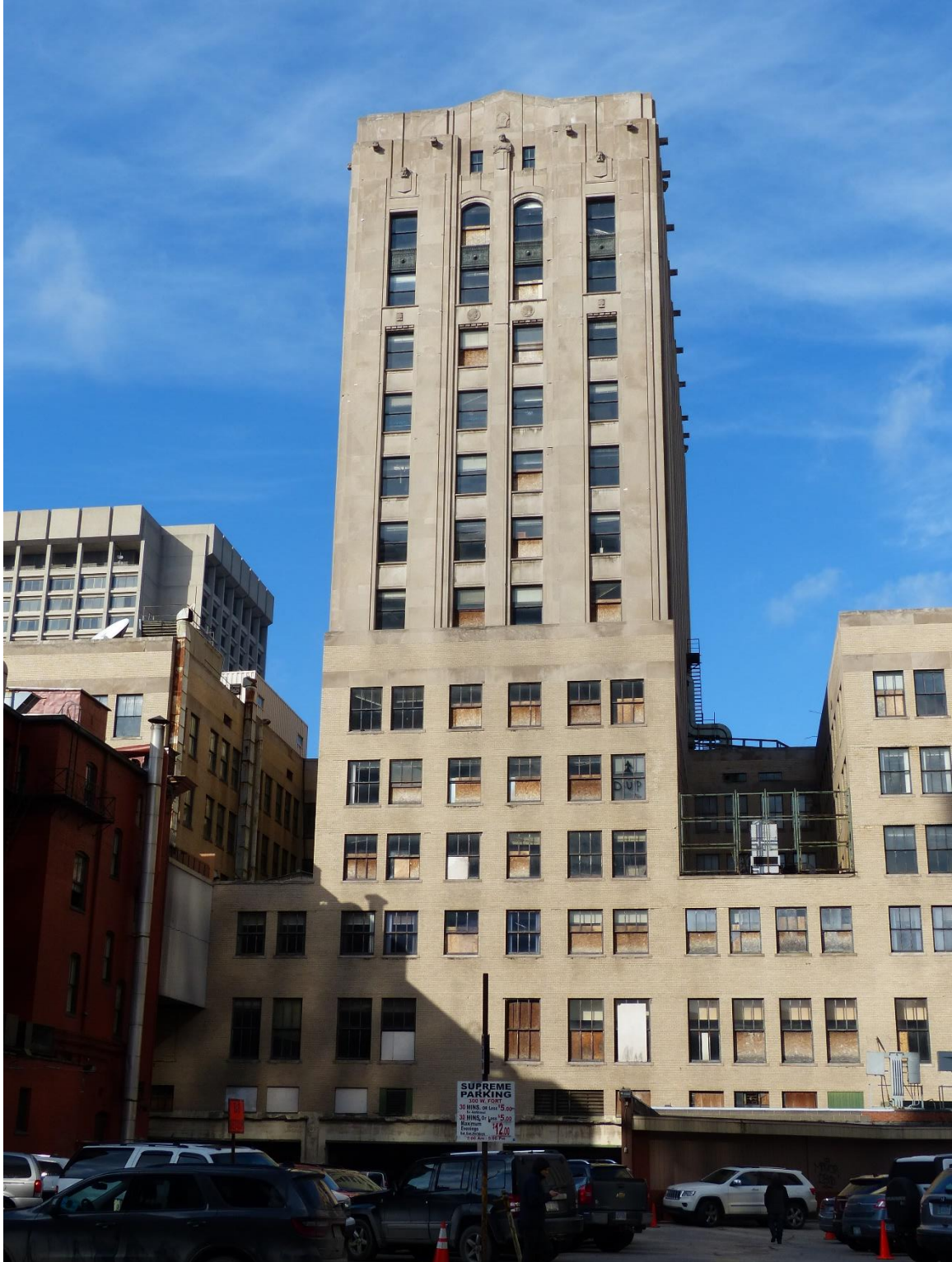
Figure #7: Exterior, Looking North. 12/7/2016
