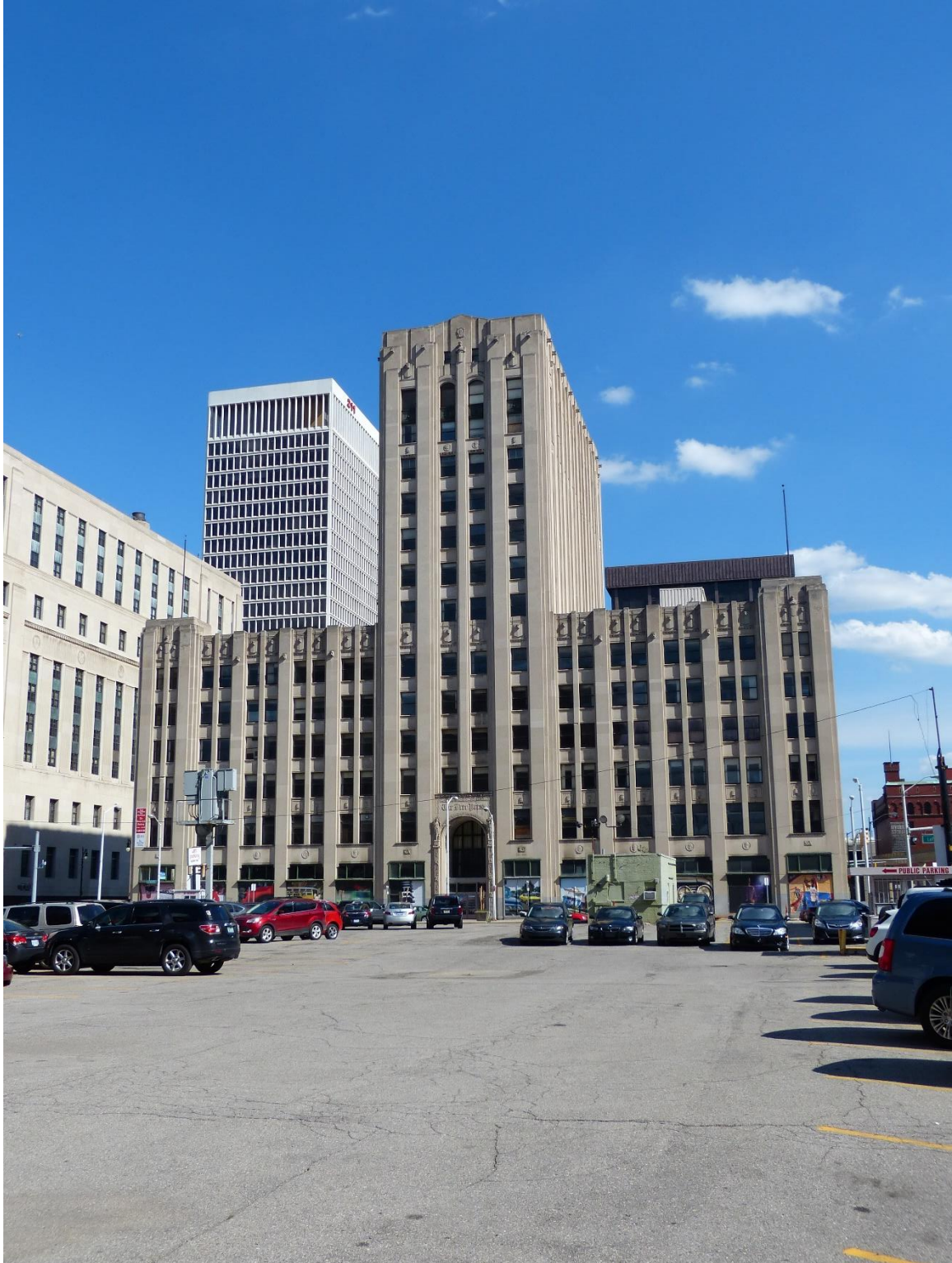
Figure #2: Exterior, Looking South. 7/25/2016
