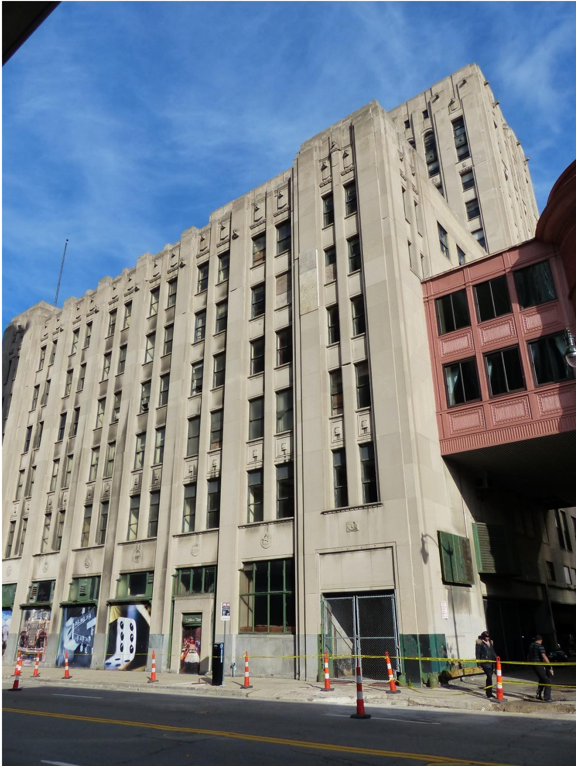
Figure #11: Exterior, Looking Northeast. 12/7/2016
