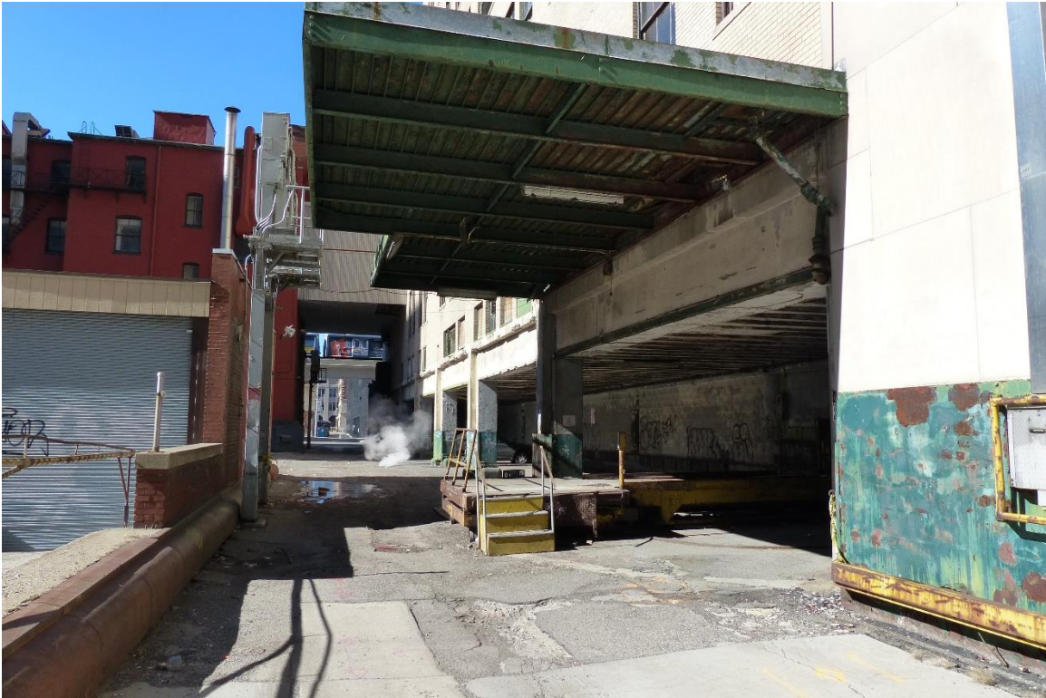
Figure #8: Exterior, Looking Northwest. 3/4/2017
