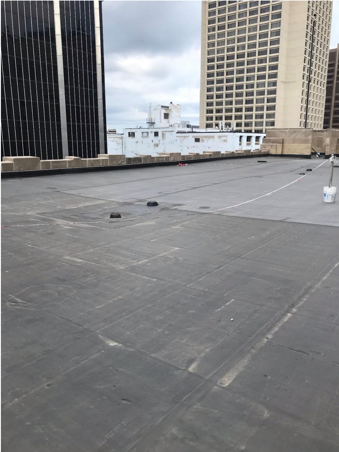
Figure #7: Exterior, West Roof, Looking Northwest. 7/31/19
