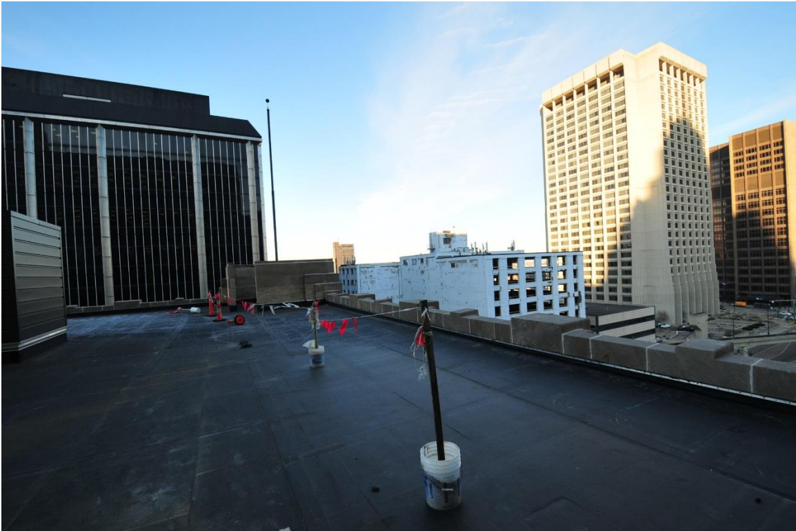
Figure #3: Exterior, West Roof, Looking Northwest. 3/11/19
