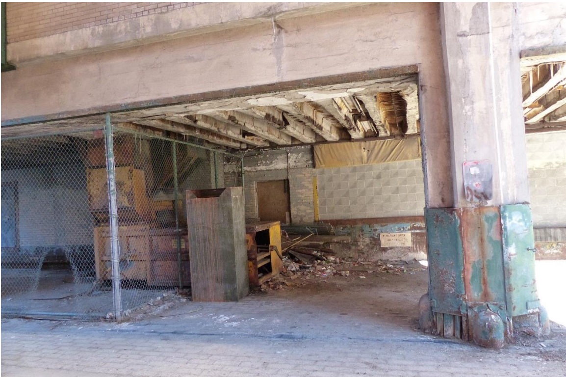
Figure #9: Exterior, Looking North. 3/4/2017
