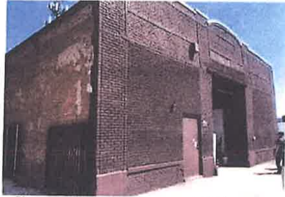
Photo 1: Looking southeast toward the subject building.
