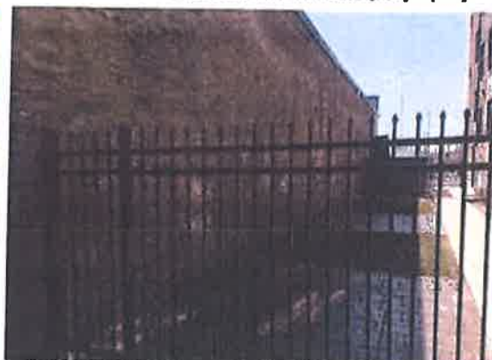
Photo 4: A view of the north side of the subject property.
