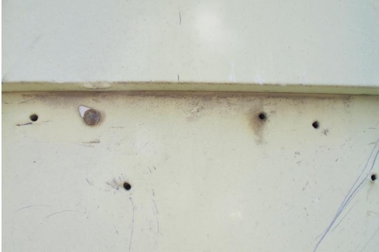
Deteriorated caulking on south side, similar across exterior
