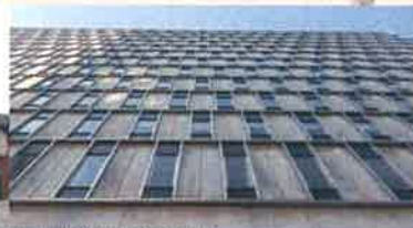
NATIONAL BANK OF DETROIT / QUBE RUNNING BOND MODULE OF WINDOWS AND MARBLE PANELS
