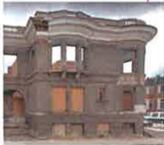
LIGHT BRICK (PATTERSON TERRACE)
