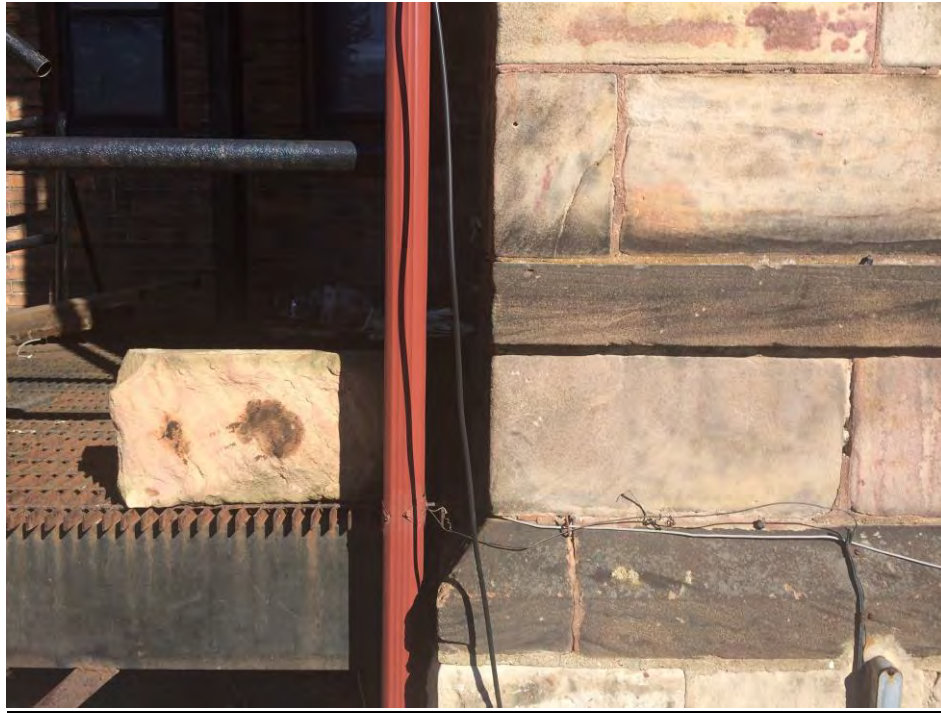
Matching sandstone to be cleaned & used for patching new door opening
