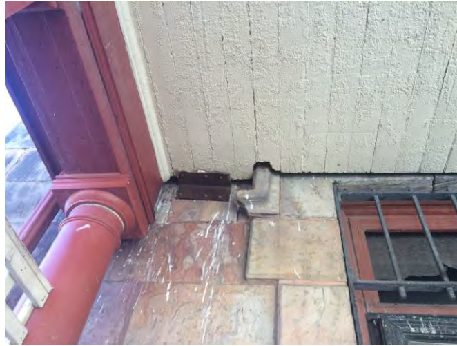
Existing wood porch ceiling top cut around sandstone details
