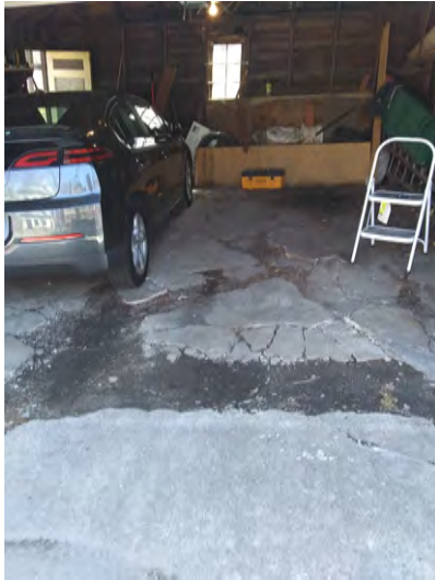
B1 CRACKED AND HEAVED GARAGE FLOOR
