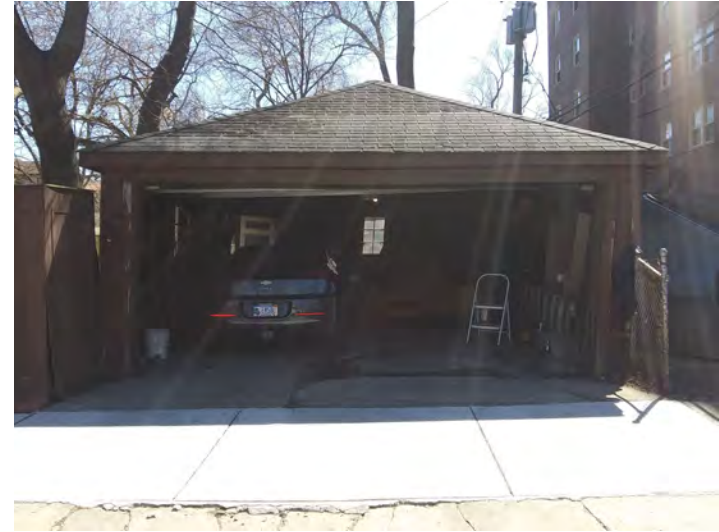
B2 — LEANING EXISTING GARAGE FRONT VIEW
