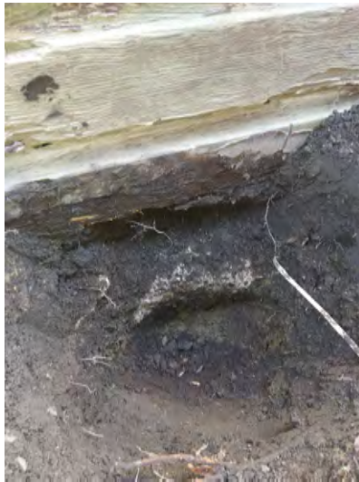
A1 — SHALLOW CONCRETE RUBBLE FOUNDATION
