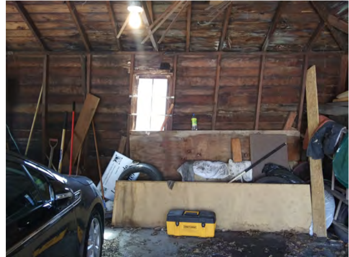
B2 CROOKED STRUCTURAL FRAME
