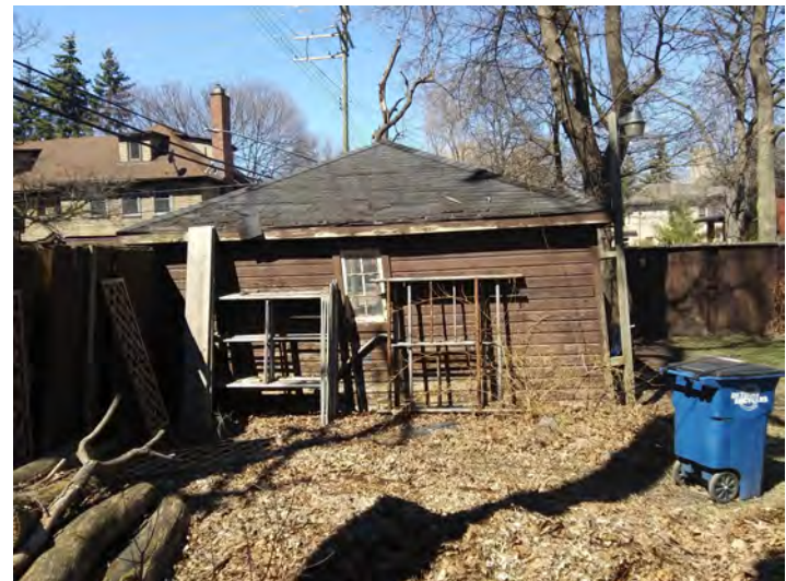
A2 SIDING AND ROOFING ARE IN POOR CONDITION
