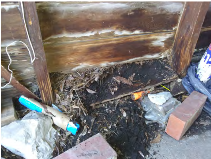
A1 STRUCTURAL DECAY AT WALL BASE
