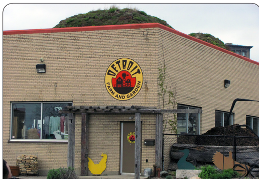
Vegetated swale in Michigan Science Center parking lot (top) green roof at Detroit Farm and Garden (bottom).
