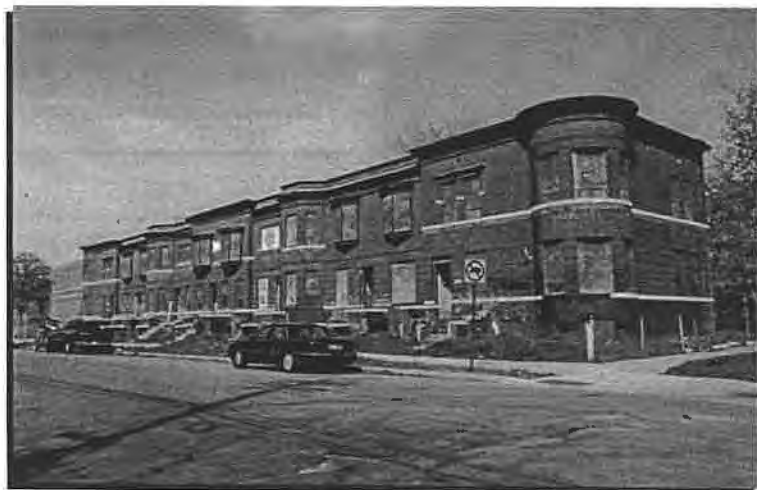
The Murray building in Southwest Detroit
