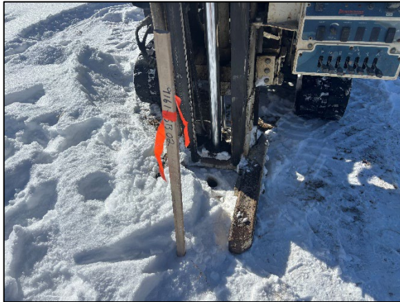
Photo 3: View of drilling 9161 SB02, facing west.
