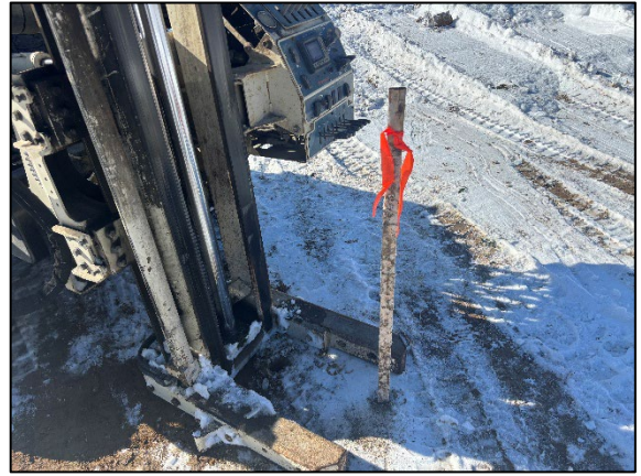
Photo 2: View of drilling at 9161 SB01, facing west.
