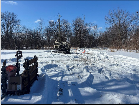
Photo 1: View of the Site pre-drilling, facing west.
