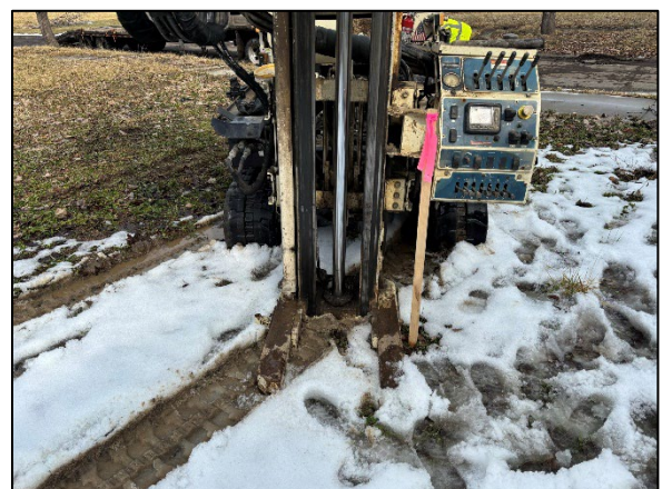
Photo 6: View of drilling at 4551 SB03, facing north.
