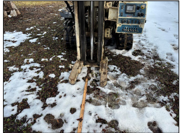
Photo 2: View of drilling at 4551 SB01, facing north.
