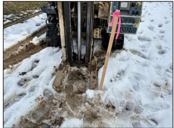
Photo 4: View of drilling at 4551 SB02, facing north.
