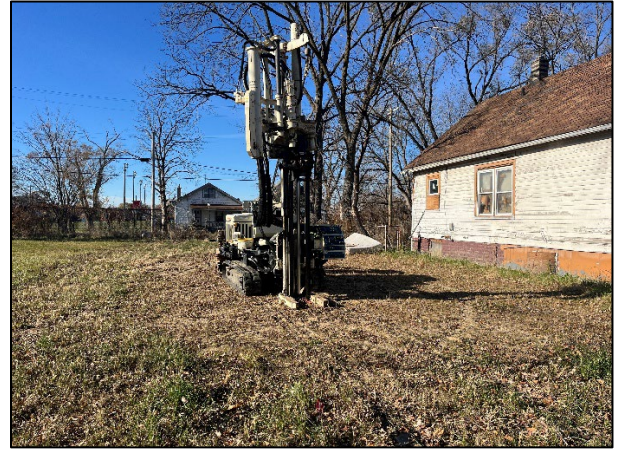
Photo 2: View of soil boring advancement
