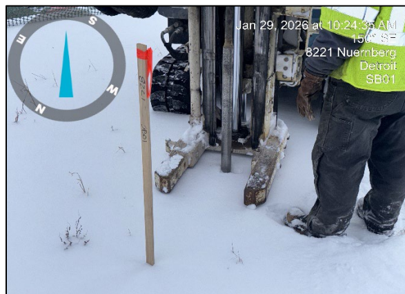
Photo 2: View of drilling at 8221 SB01, facing southeast.
