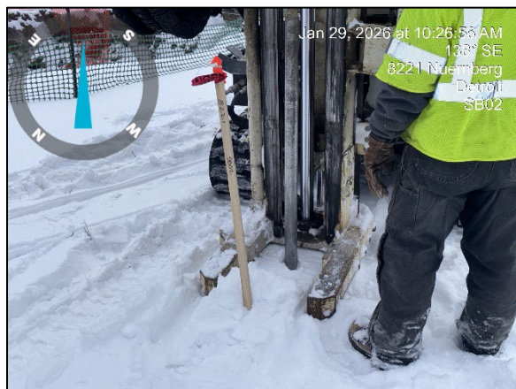
Photo 3: Viewing 8221 SB02 soil recovery, facing southeast.
