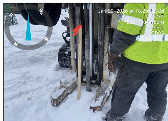
Photo 4: View of drilling at 8221 SB03, facing southeast.
