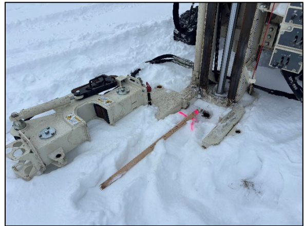
Photo 4: View of drilling at 8192 SB02, facing southeast.
