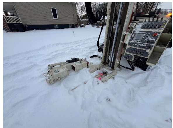
Photo 6: View of drilling at 8192 SB03, facing southeast.
