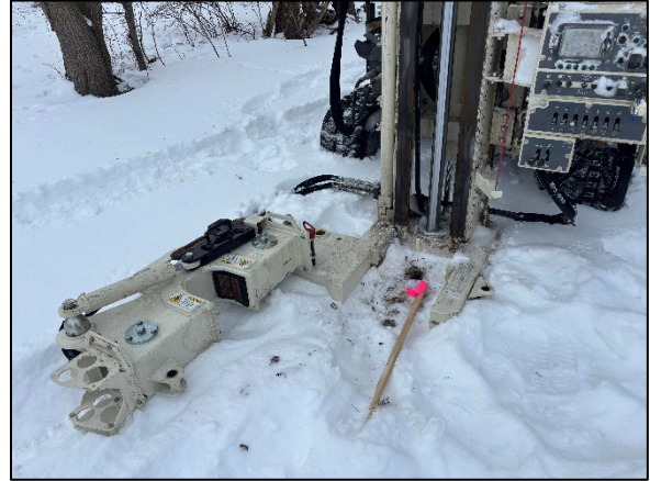
Photo 2: View of drilling at 8192 SB01, facing southeast.
