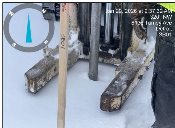
Photo 2: View of drilling at 8136 SB01, facing northwest.
