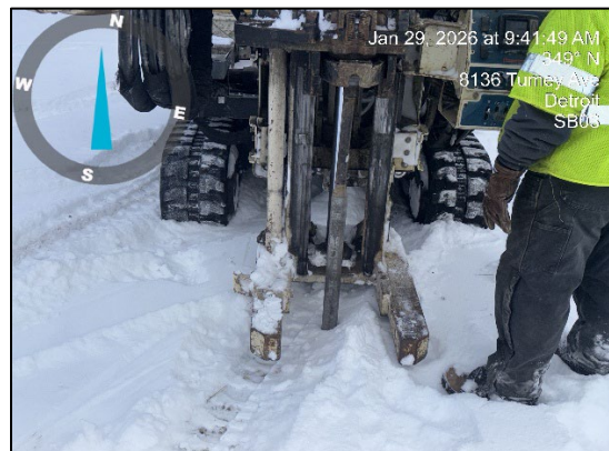
Photo 4: View of drilling at 8136 SB03, facing north.
