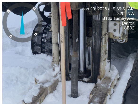
Photo 3: View of drilling 8136 SB02, facing northwest.
