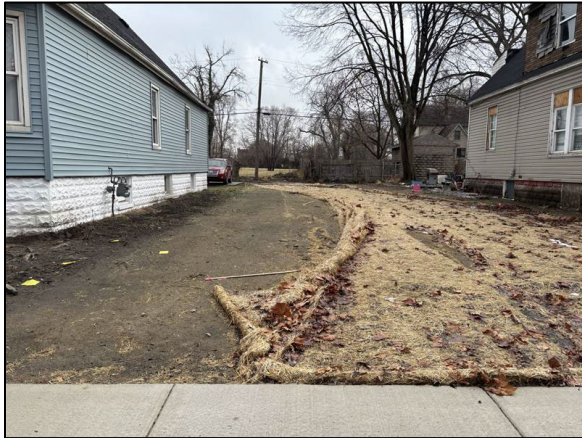
Photo 1: View of the Site pre-drilling, facing southeast.
