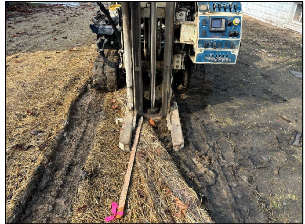
Photo 2: View of drilling at 8087 SB01, facing northwest.
