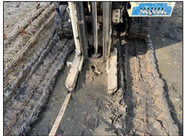
Photo 4: View of drilling at 8087 SB02, facing northwest.
