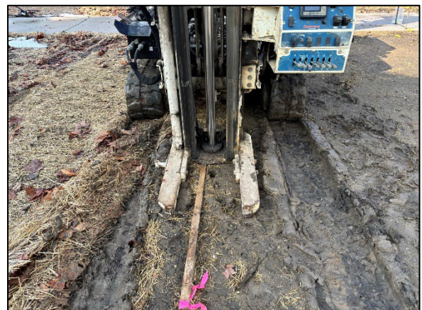
Photo 6: View of drilling at 8087 SB03, facing northwest.
