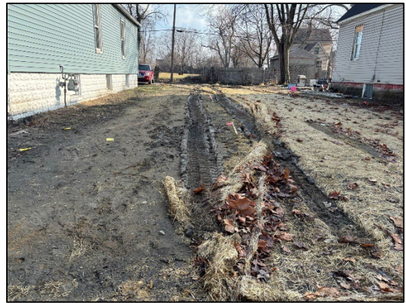
Photo 8: View of the Site post-drilling, facing southeast.
