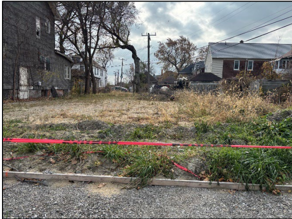
Photo 1: Viewing Site Pre-Drilling, Facing South.
