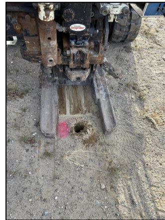
Photo 4: Viewing 7532 SB02 Drilling, Facing South.
