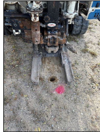
Photo 2: Viewing 7532 SB01 Drilling, Facing South.
