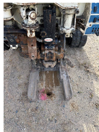
Photo 6: Viewing 7532 SB03 Drilling, Facing South.
