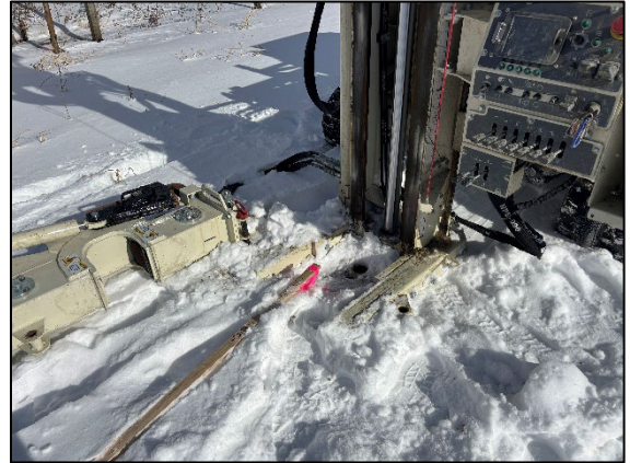
Photo 2: View of 6658 SB01, facing northeast.
