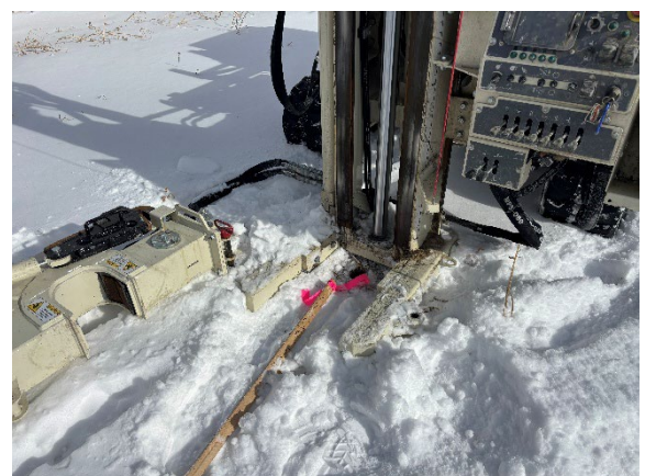
Photo 6: View of 6658 SB03, facing northeast.
