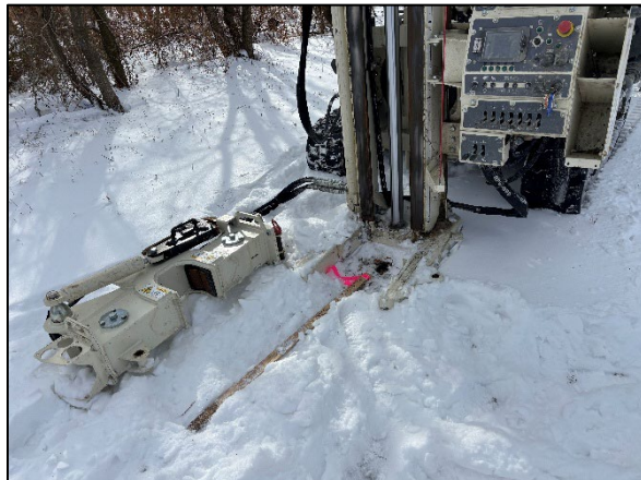
Photo 4: View of 6451 SB02, facing south.
