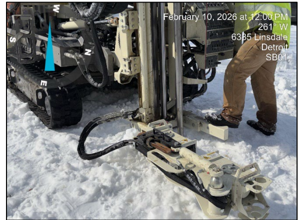
Photo 2: View of drilling at 6385 SB01, facing west.
