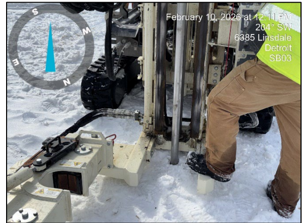
Photo 4: View of drilling at 6385 SB03, facing southwest.
