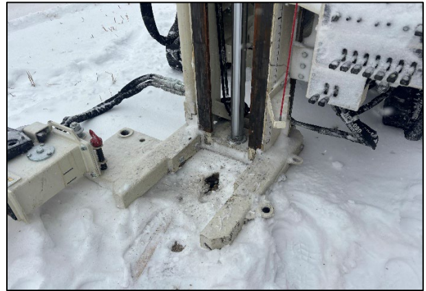
Photo 2: View of drilling at 5971 SB01, facing northeast.
