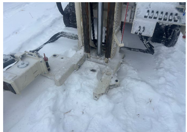
Photo 6: View of drilling at 5971 SB03, facing northeast.
