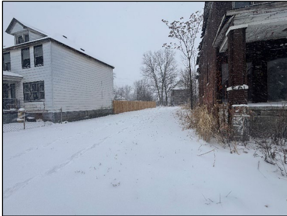
Photo 1: View of the Site pre-drilling, facing northeast.
