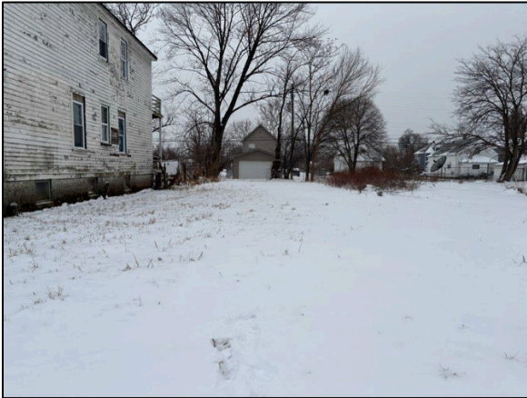
Photo 1: View of the Site pre-drilling, facing southwest.
