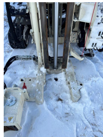
Photo 6: View of drilling at 5785 SB03, facing southwest.
