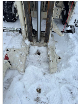
Photo 4: View of drilling at 5785 SB02, facing southwest.
