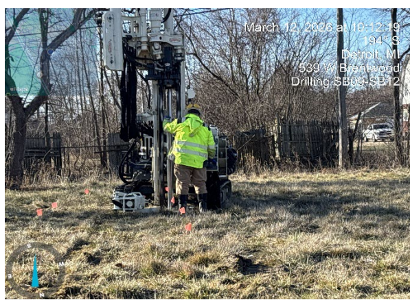
Photo 6: View of drilling at 539 SB09 – SB12, facing south.
