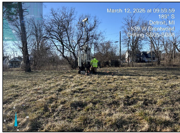
Photo 4: View of drilling at 539 SB05 - SB08, facing south.
