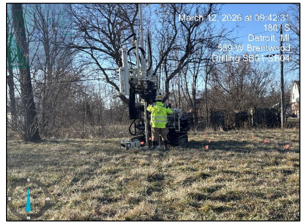
Photo 2: View of drilling at 539 SB01 – SB04, facing south.
