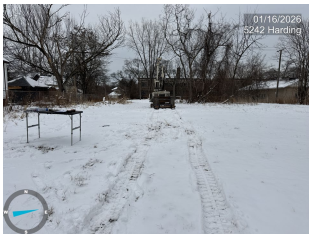
Photo 3: View of the Site pre-drilling, facing east.
