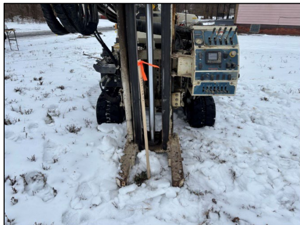
Photo 4: View of drilling at 3999 SB02, facing south.
