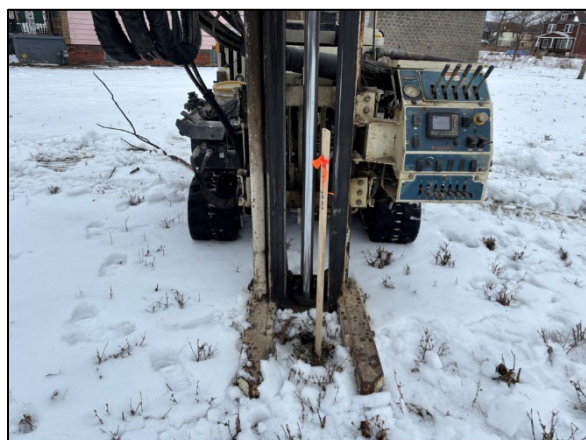
Photo 6: View of drilling at 3999 SB03, facing south.
