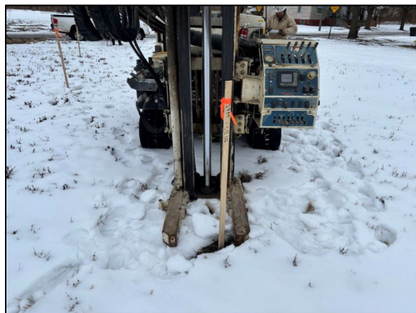
Photo 2: View of drilling at 3999 SB01, facing east.
