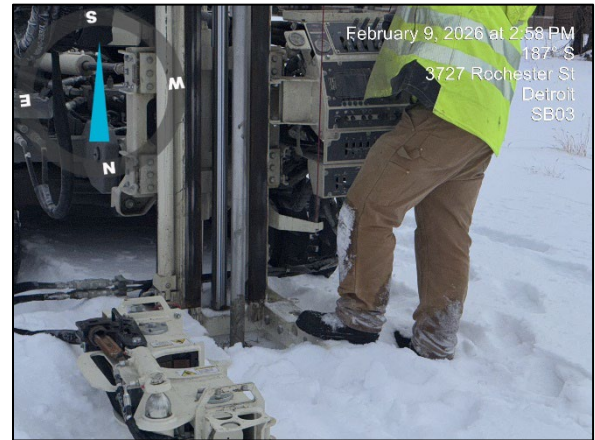
Photo 4: View of drilling at 3727 SB03, facing south.
