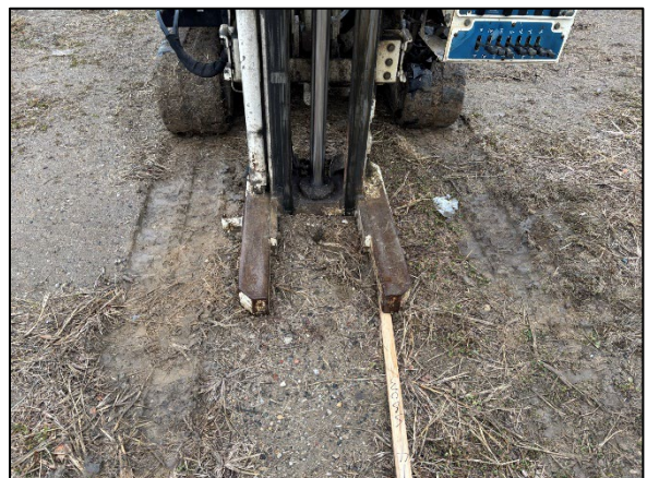
Photo 6: View of drilling at 3314 SB03, facing southeast.
