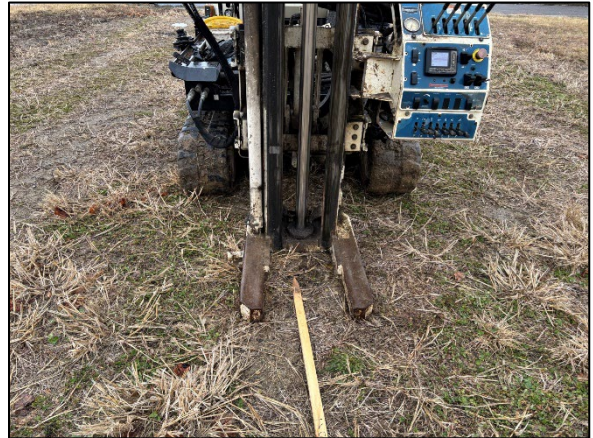
Photo 2: View of drilling at 3314 SB01, facing southeast.
