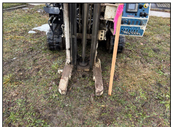
Photo 6: View of drilling at 2257 SB03, facing northwest.
