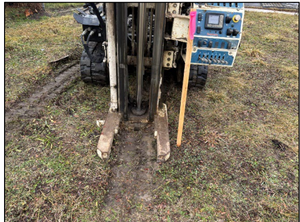
Photo 4: View of drilling at 2257 SB02, facing northwest.
