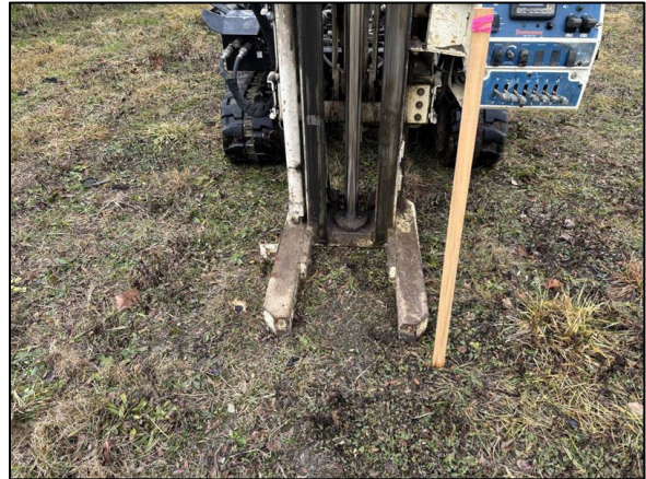
Photo 2: View of drilling at 2257 SB01, facing northwest.
