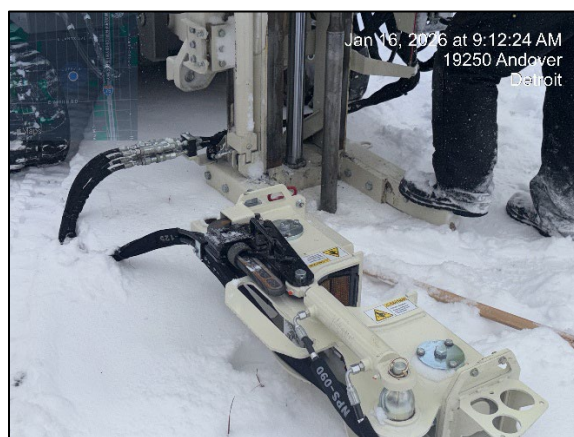
Photo 2: View of drilling at 19250 SB01, facing east.
