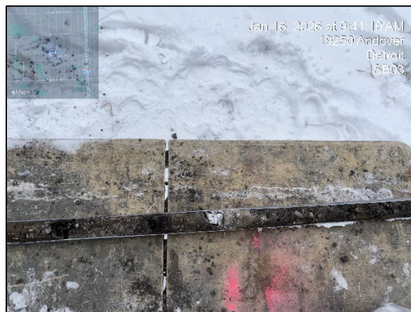
Photo 4: View of drilling at 19250 SB03, facing east.
