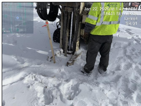
Photo 3: Viewing drilling at 18441 SB01, facing northeast.
