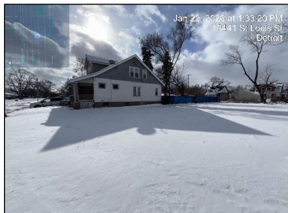
Photo 2: View of the Site pre-drilling, facing northeast.
