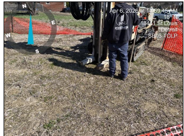
Photo 10: View of drilling at 18441 SB03 TCLP, facing north.
