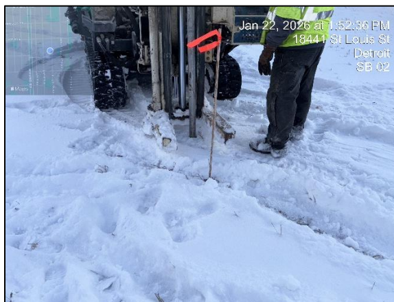
Photo 4: View of drilling at 18441 SB02, facing northeast.
