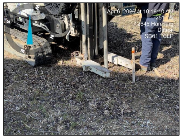
Photo 7: View of drilling at 12645 TCLP SB01, facing west.
