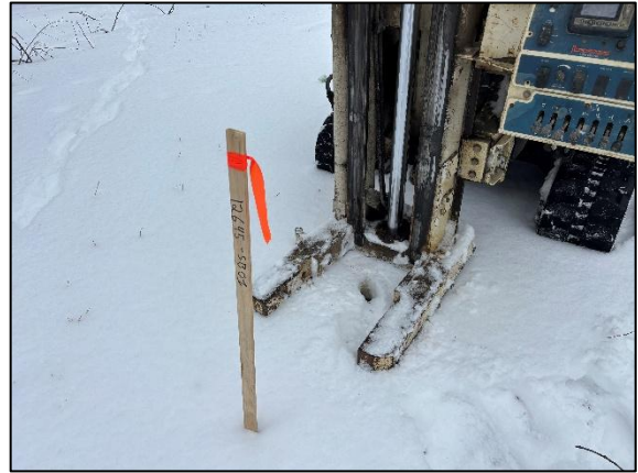
Photo 2: View of drilling at 12645 SB01, facing north.
