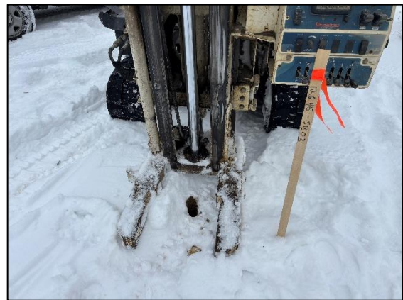
Photo 4: View of drilling at 12645 SB03, facing north.
