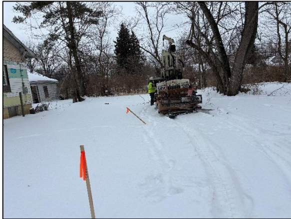
Photo 1: View of the Site pre-drilling, facing southwest.
