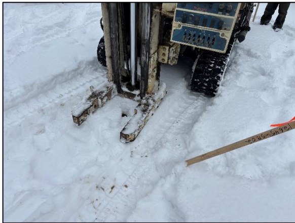
Photo 3: View of drilling 12645 SB02, facing north.
