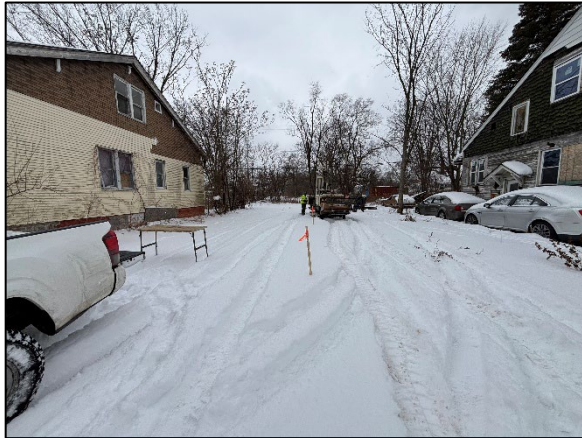
Photo 1: View of the Site pre-drilling, facing southwest.
