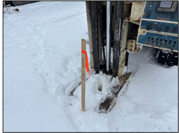
Photo 2: View of drilling at 12643 SB01, facing north.
