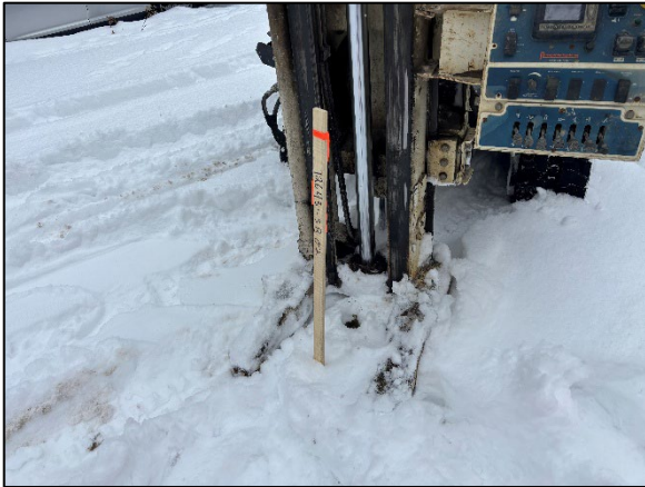
Photo 3: View of drilling 12643 SB02, facing north.
