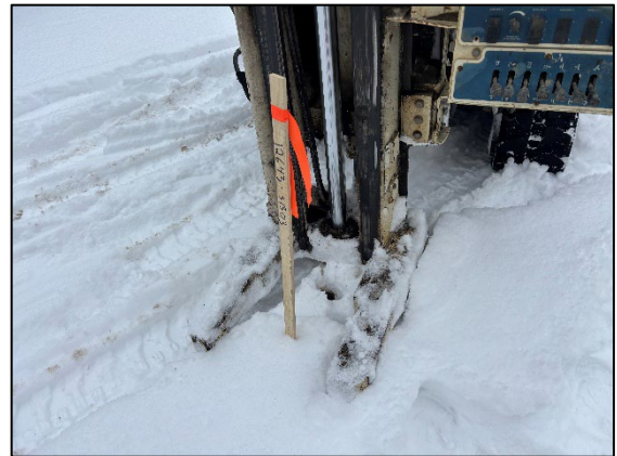
Photo 4: View of drilling at 12643 SB03, facing north.
