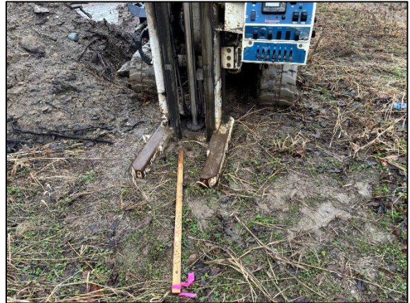
Photo 2: View of drilling at 1230 SB01, facing southeast.
