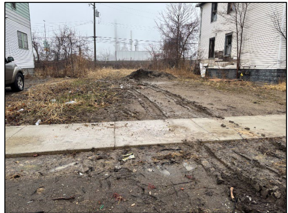
Photo 8: View of the Site post-drilling, facing northwest.
