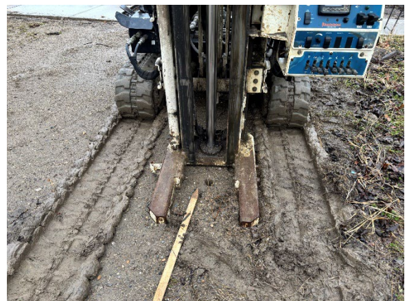
Photo 6: View of drilling at 1230 SB03, facing southeast.
