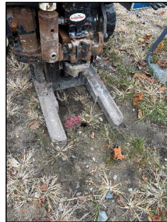
Photo 4: Viewing 12275 SB02 Drilling, Facing Northwest.
