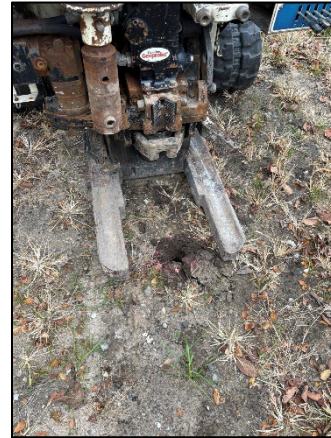
Photo 2: Viewing 12275 SB01 Drilling, Facing Northwest.
