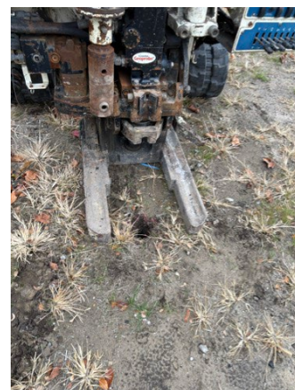
Photo 6: Viewing 12275 SB03 Drilling, Facing Northwest.
