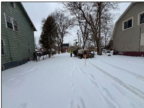
Photo 1: View of the Site pre-drilling, facing north.
