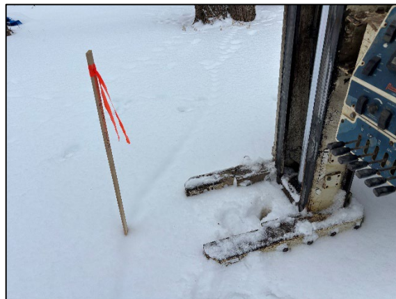
Photo 2: View of drilling at 12145 SB01, facing east.
