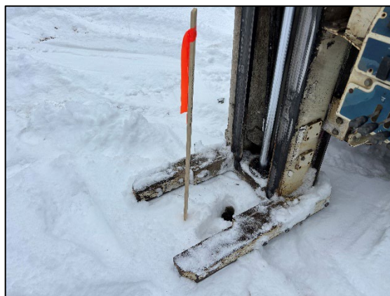
Photo 4: View of drilling at 12145 SB03, facing east.
