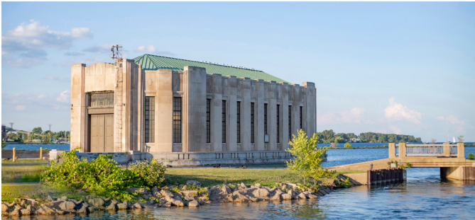
GLWA Belle Isle intake station
