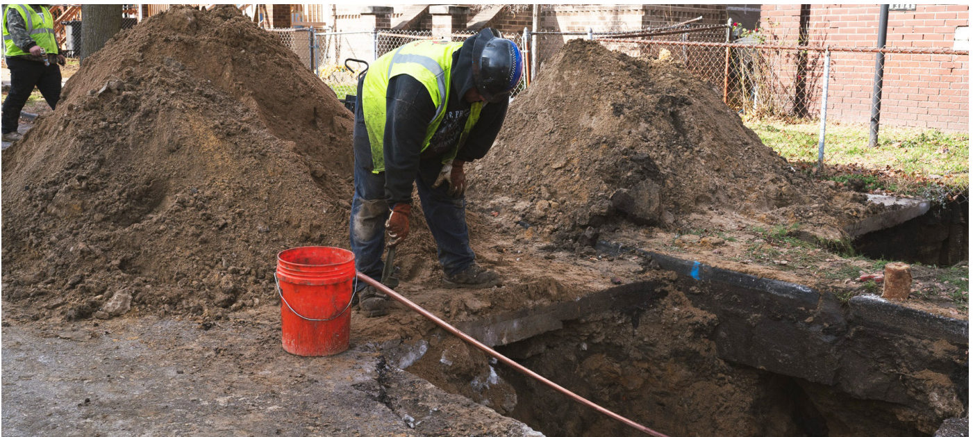
A DWSD contractor replaces a lead service line with copper.
