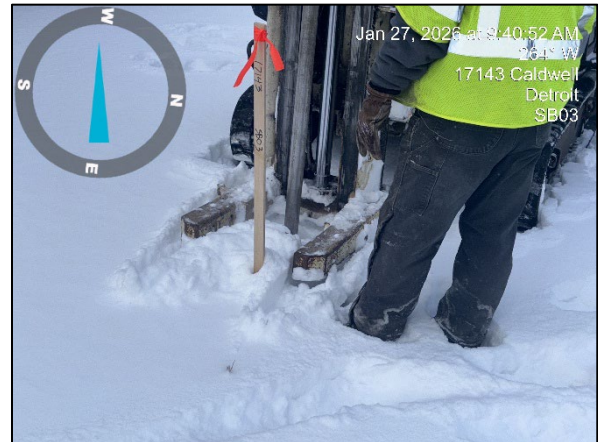
Photo 4: View of drilling at 17143 SB03, facing west.
