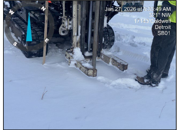
Photo 2: View of drilling at 17143 SB01, facing northwest.
