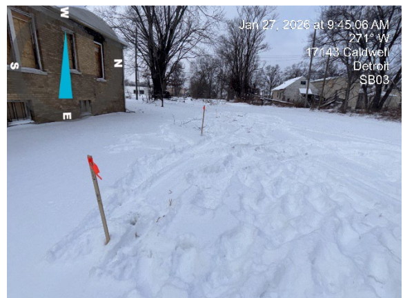
Photo 6: View of the site post-drilling, facing west
