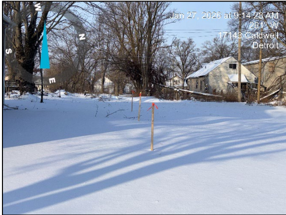
Photo 1: View of the Site pre-drilling, facing west.
