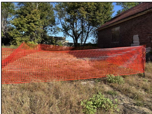
Photo 11:View of Site at the time of TCLP soil boring activities
