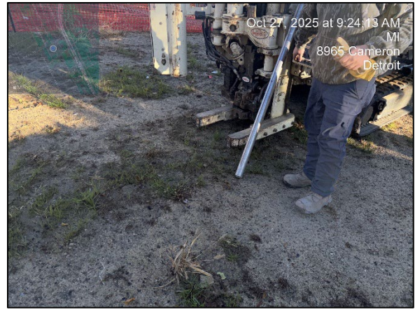
Photo 14: Viewing boring location at the time of supplemental soil sampling activities
