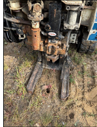
Photo 2: Viewing 8649 SB01 Drilling, Facing North.
