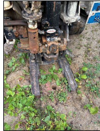
Photo 4: Viewing 8649 SB02 Drilling, Facing North.
