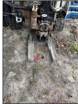
Photo 4: Viewing 5928 SB02 Drilling, Facing Northeast.
