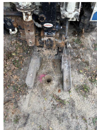
Photo 6: Viewing 5928 SB03 Drilling, Facing Northeast.
