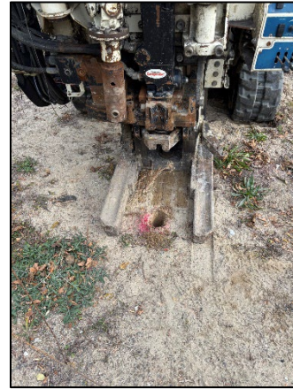
Photo 2: Viewing 5928 SB01 Drilling, Facing Northeast.
