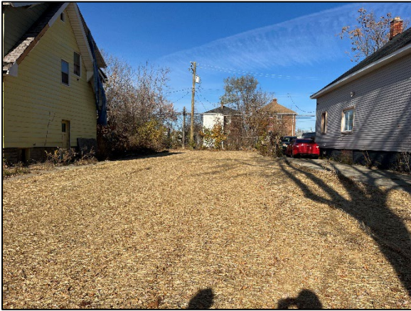
Photo 1: View of Site pre-drilling
