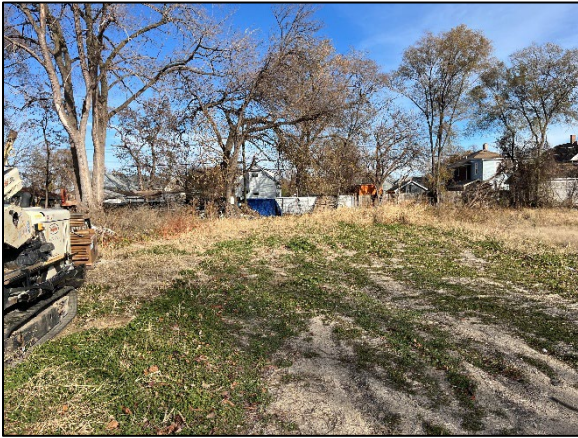
Photo 1: View of Site pre-drilling
