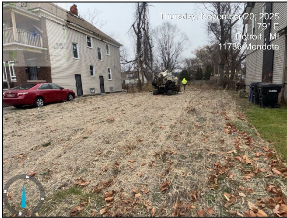
Photo 1: View of Site pre-drilling
