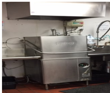
Type II hood over heat/moisture producing dishmachine
