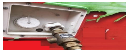
Backflow preventer installed on exterior of unit for connection of public water line
