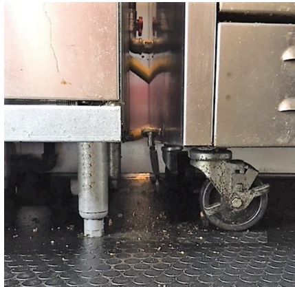
Floor mounted equipment elevated on 6-inch legs or on castors to move for cleaning.
