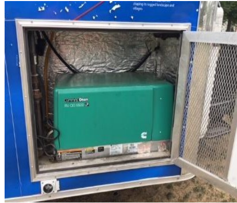
Generator installed in exterior compartment of unit
