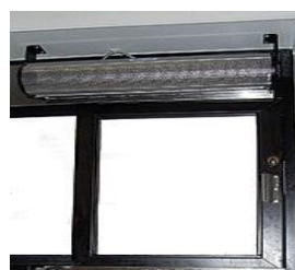
Air curtain over pass through window
