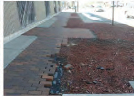
C Failed paving and bare planting beds on Livernois south of 7 Mile.
