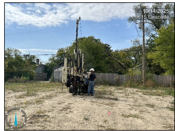
Photo 4: Viewing advancement of 9615 Cascade SB-3
