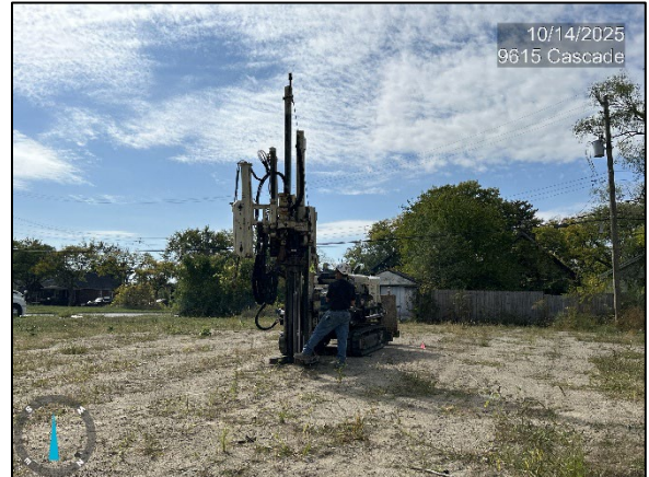
Photo 2: Viewing advancement of 9615 Cascade SB-1
