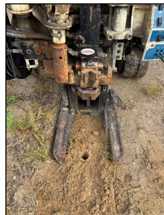
Photo 6: Viewing 8649 SB03 Drilling, Facing North.
