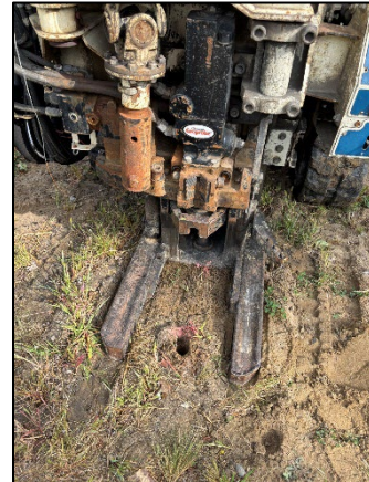
Photo 2: Viewing 8649 SB01 Drilling, Facing North.
