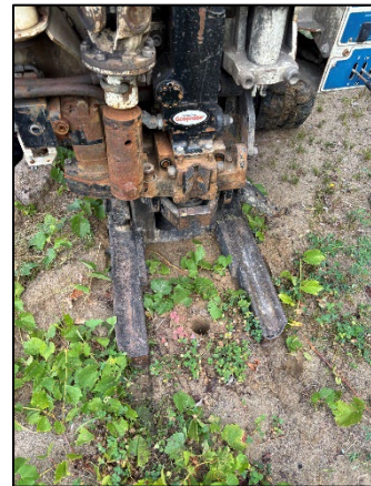
Photo 4: Viewing 8649 SB02 Drilling, Facing North.
