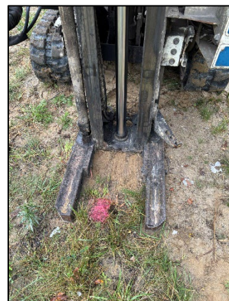
Photo 6: Viewing 8221 SB03 Drilling, Facing North.
