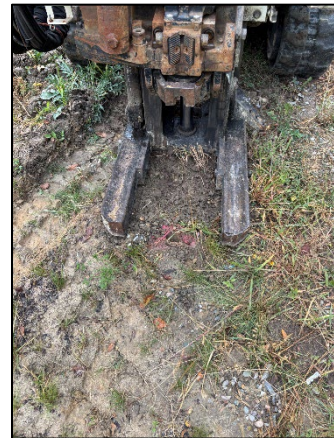
Photo 4: Viewing 8221 SB02 Drilling, Facing North.
