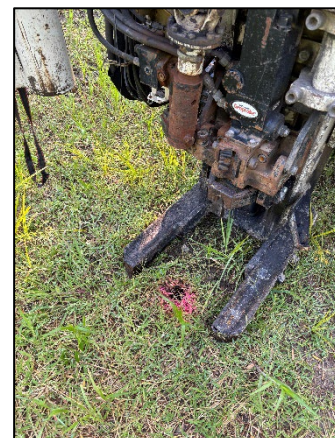
Photo 6: Viewing 8121 SB03 Drilling, Facing West.
