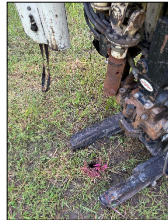
Photo 4: Viewing 8121 SB02 Drilling, Facing West.
