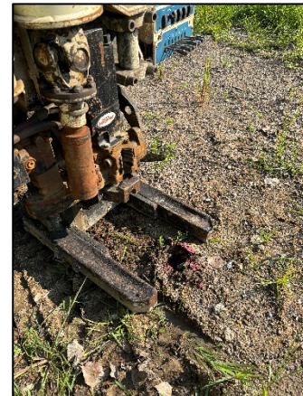
Photo 4: Viewing 8070 SB02 Drilling, Facing East.
