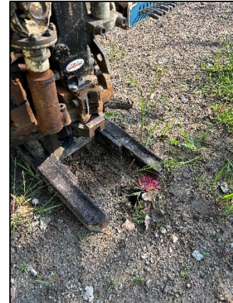
Photo 2: Viewing 8070 SB01 Drilling, Facing East.
