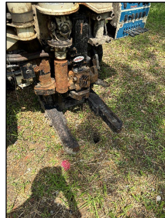
Photo 2: Viewing 14404 SB01 Drilling, Facing Northeast.
