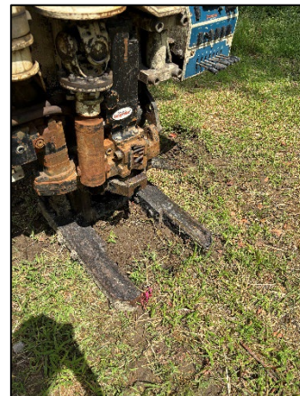
Photo 4: Viewing 14404 SB02 Drilling, Facing Northeast.
